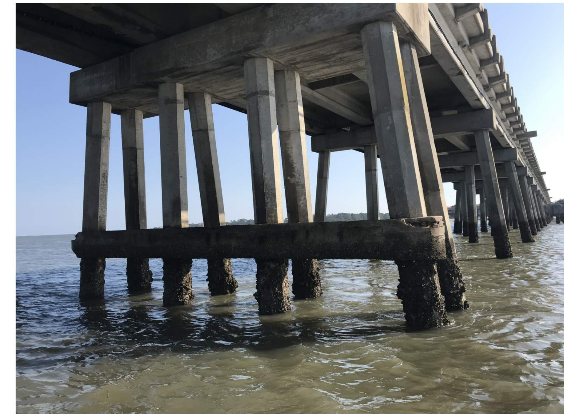
PHOTO 2: TYPICAL COLLAR ELEVATION
