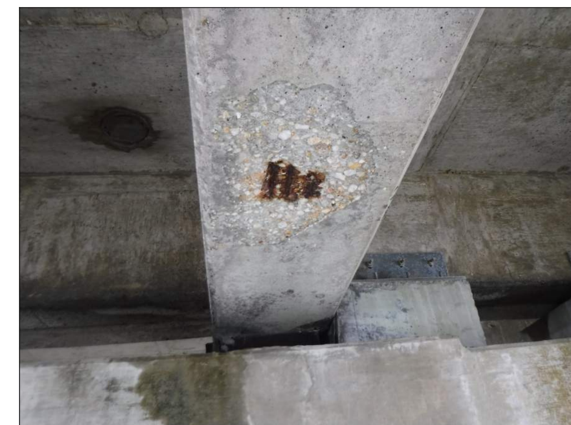
PHOTO 2: TYPICAL SPALL REPAIR ITEM
